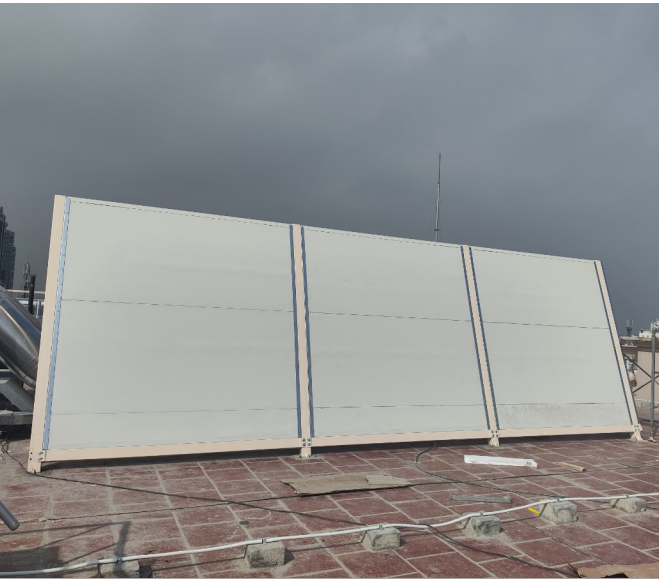
Masterise Hang Bai - Noise Barriers on Rooftop
