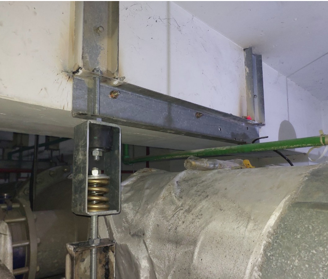
Sarimi Office HCMC - Anti-vibration System
